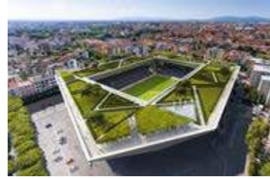
16 Redesign of the Stadium Arena Garibaldi, Pisa (I)
