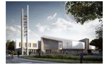
43 New Varignano Parish Centre, Viareggio (I)
