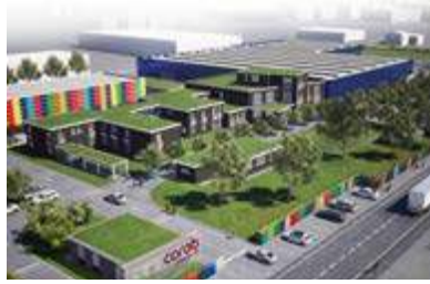
13 Refurbishment and expansion of Corob plant, S. Felice sul Panaro (I)
