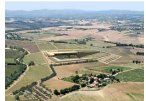
103 New Municipal Stadium, Siena (I)
